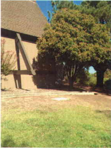
View looking towards radio cabinet south of the Church. Cabinet is well screened.
