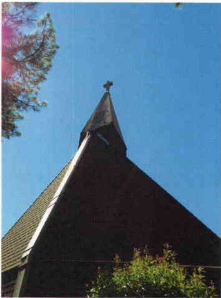
Close up view of T-Mobile steeple structure
