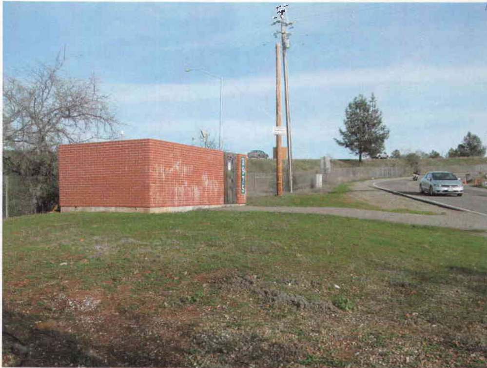
Top – MetroPCS 10' x 20' ground space / equipment cabinet enclosure with 6' tall CMU brick wall Below: Location within existing enclosure for third equipment cabinet.
