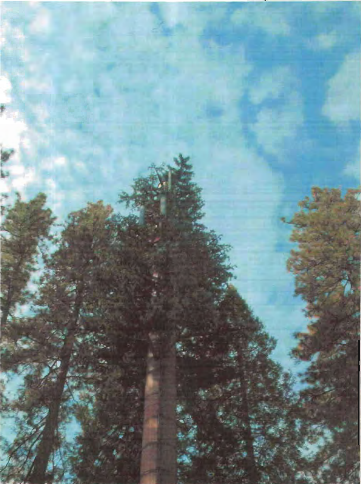
PHOTO OF TREE TOP SHOWING PAINTED ANTENNAS
