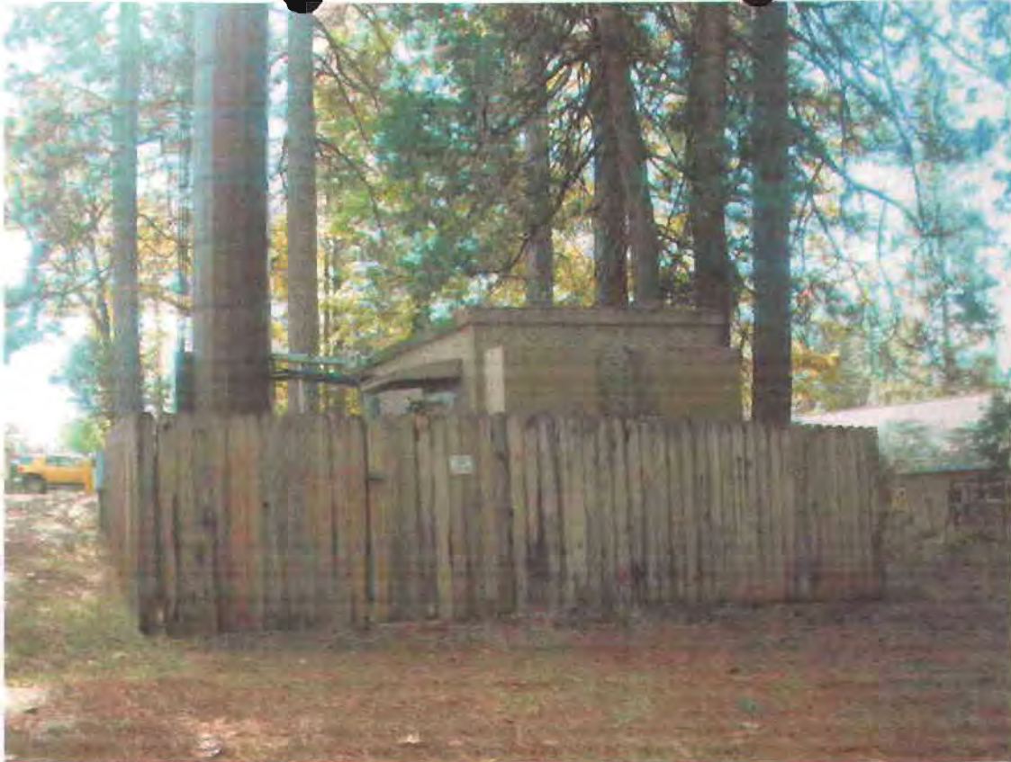
PHOTO OF T-MOBILE SHELTER AND FENCING
