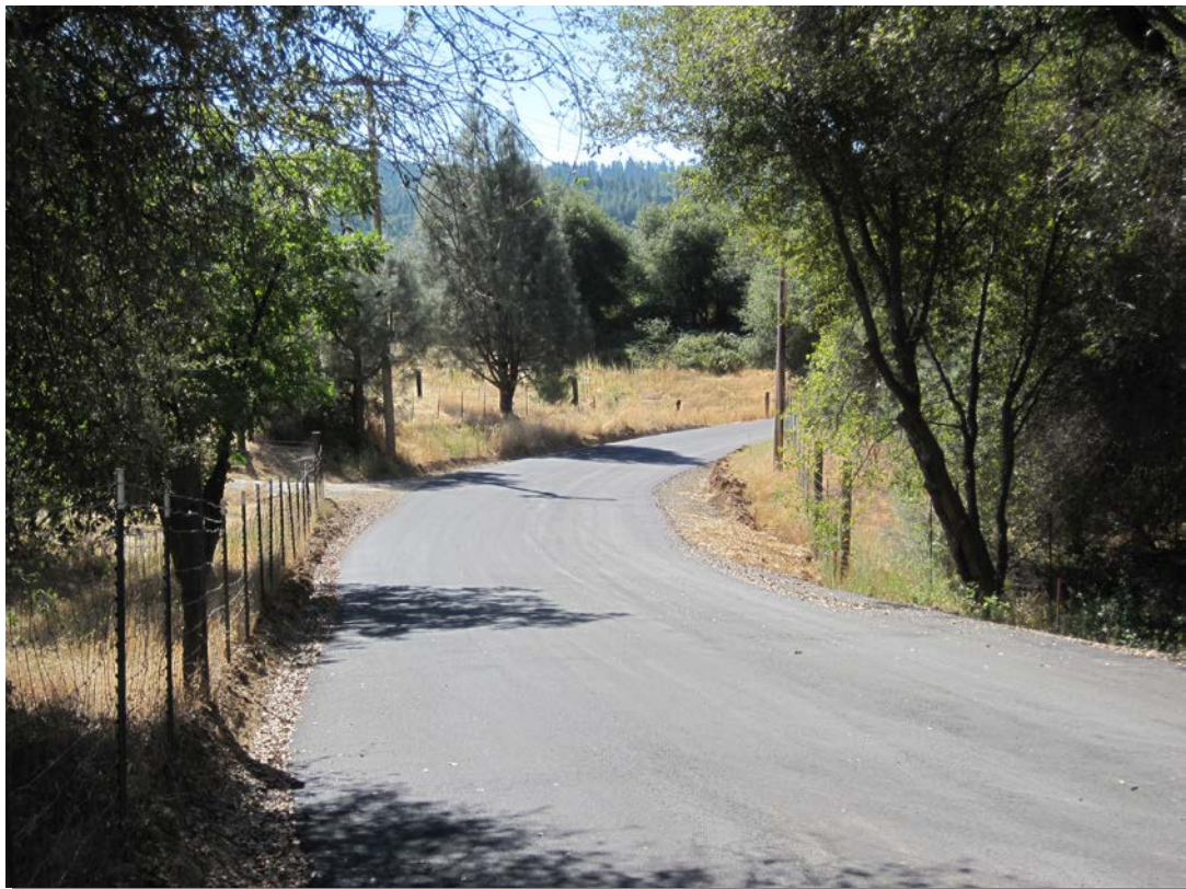
Newly paved private road accessing winery
